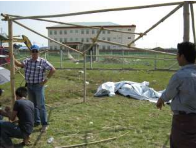
Frame complete and ready for tarpaulin attachment
