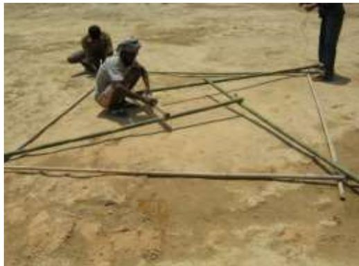
Complete RSK roof frame is assembled on the ground
