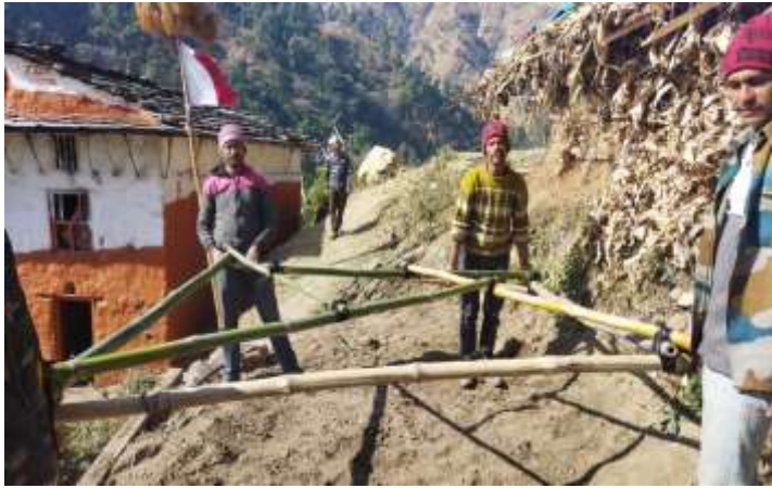
Carrying the roof frame to shelter site
