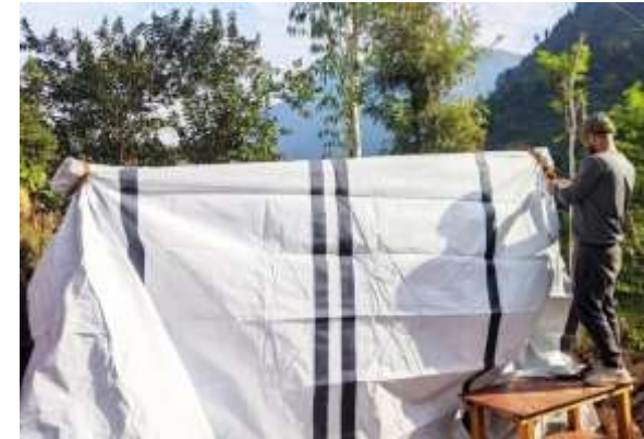
Shelter 6 (family of 4 ) Nearing completion
