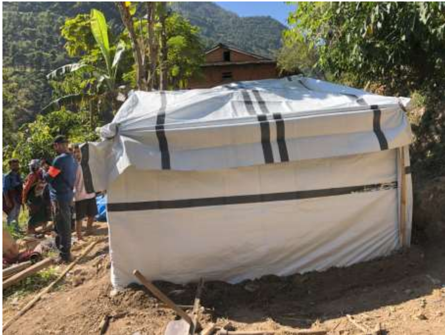
First shelter (family of 6 ) nears completion.
