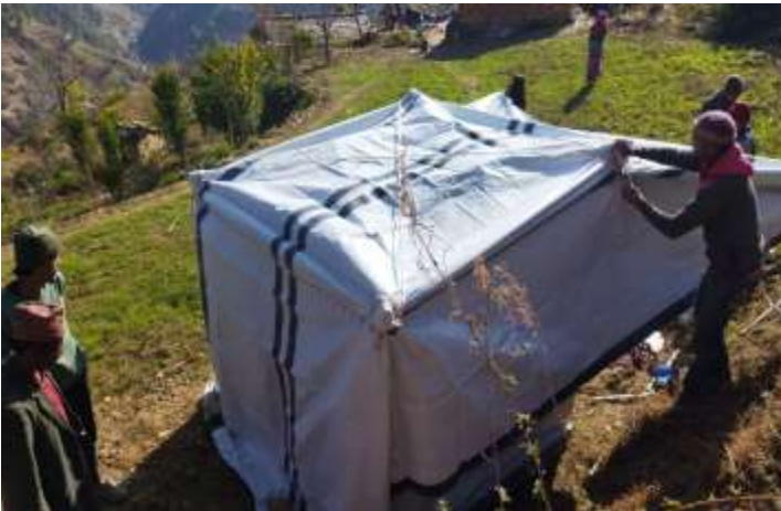
Building the reduced internal volume RSK shelter
