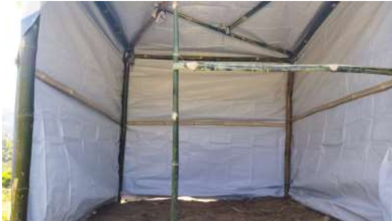
Inside of an RSK shelter being built
