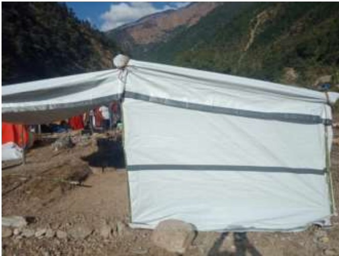
The shelters were built to a good standard
