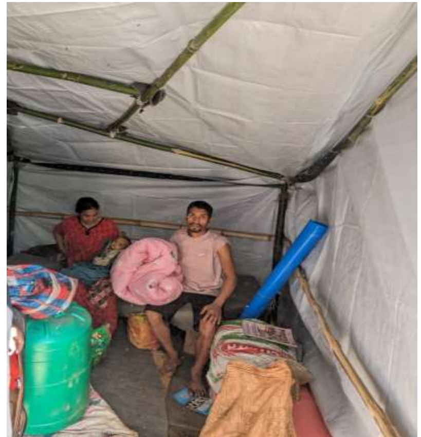
Mats on the ground for insulation as the first RSK shelter nears completion.
