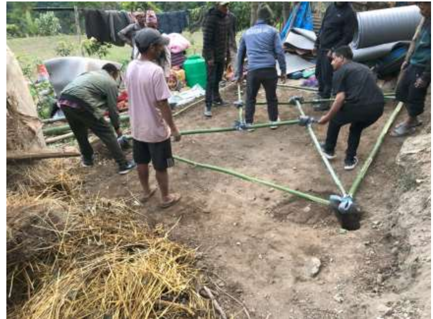
Digging the holes for the RSK four corner posts.
