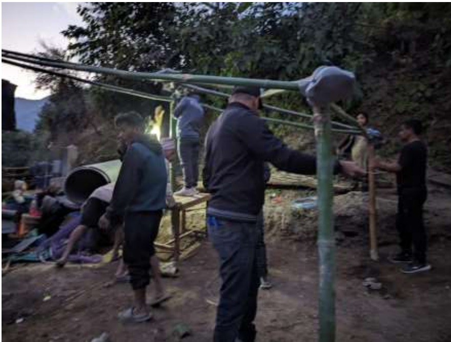
First RSK shelter being erected by lamp light.
