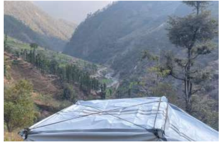
The roof frame in position
