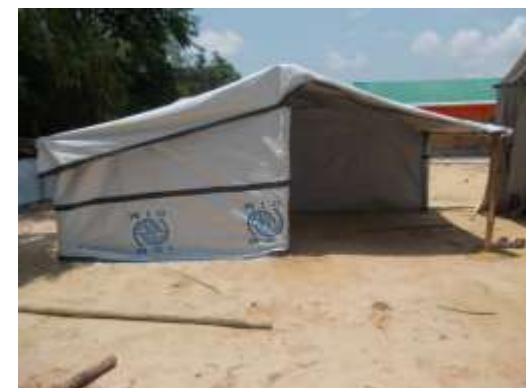
Walls are filled in with tarpaulins or bamboo lattice
