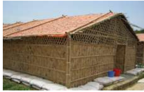
Traditional roof hospital. Photo. S.Halbert May 2018
