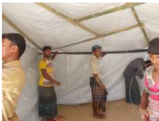
Final fitting of tarpaulin inside shelter
