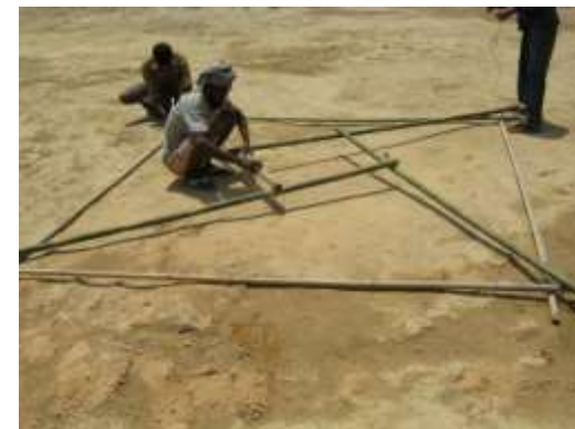
Simple assembly of roof frame on the ground
