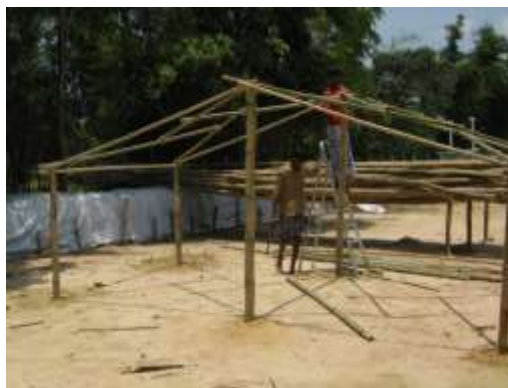
Shelter frame complete
