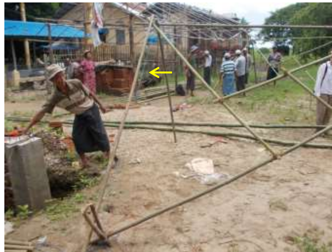
side rope (arrowed) being replaced by bamboo
