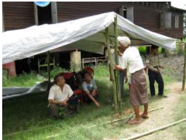
Second central support post in position
