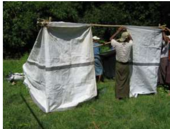
Front tarpaulin opening secured
