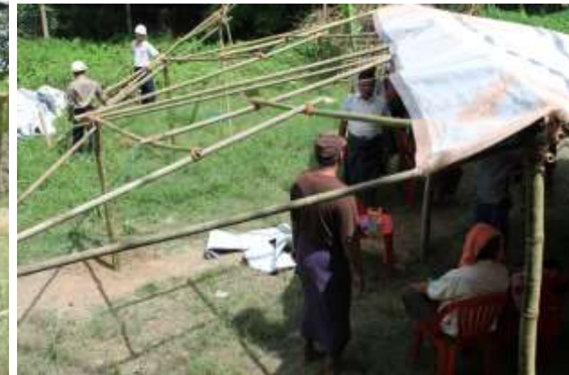
4 unit frame nears completion
