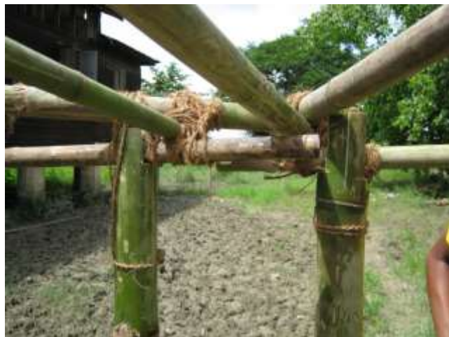
Standard arrangement. Side ridge poles secured on top of main support ridge poles
