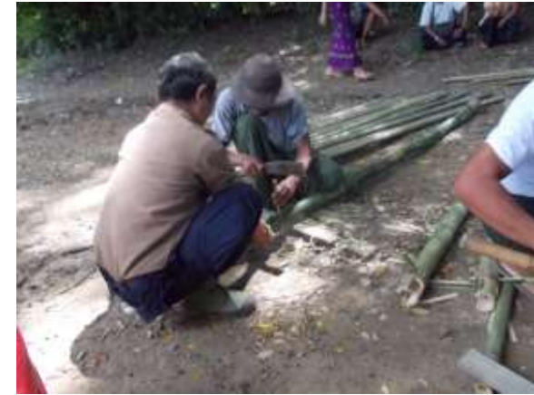
Cutting the dowel holes on the posts
