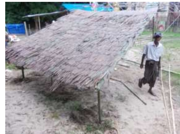
Elevated roof shelter. If slightly higher (3 feet) lower support posts had been used, this would have enabled the shelter to be lowered to the ground at the upper ridge pole and thereby provide the additional severe storm security of the storm profile shelter.
