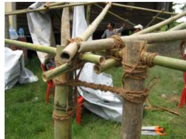
Alternative arrangement. Side ridge poles secured beneath main support ridge poles
