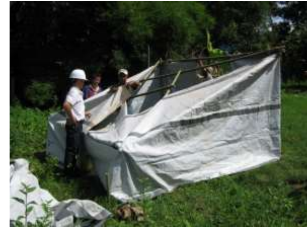
Two half tarpaulins positioned and being attached to central roof frame
