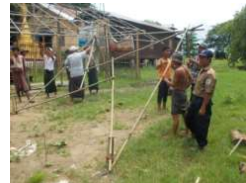
both side ropes replaced by poles
