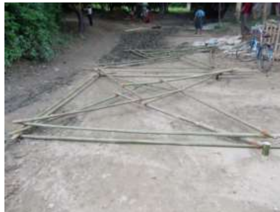
Classroom frames ready for moving
