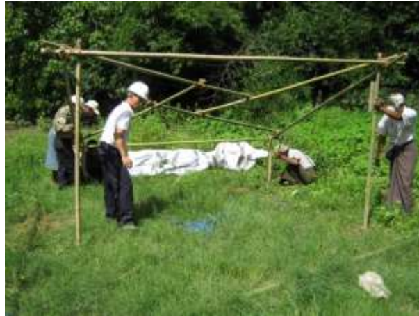
Single elevated frame 12 pole frame
