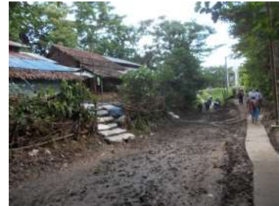
Flood defences ineffective for flooding over 6 feet
