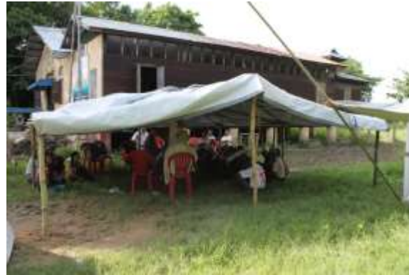
The complete shelter awaiting wall construction
