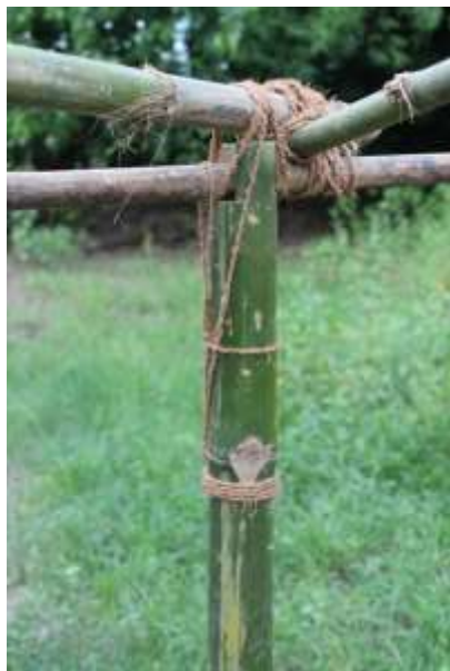
Tie down arrangement below bamboo node
