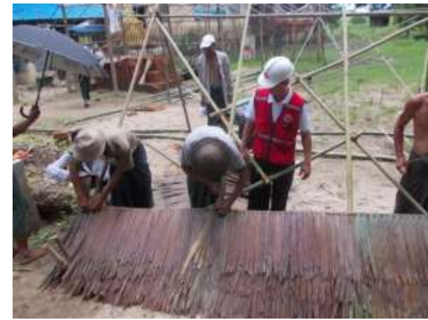
Two lengths of split bamboo provide the required support
