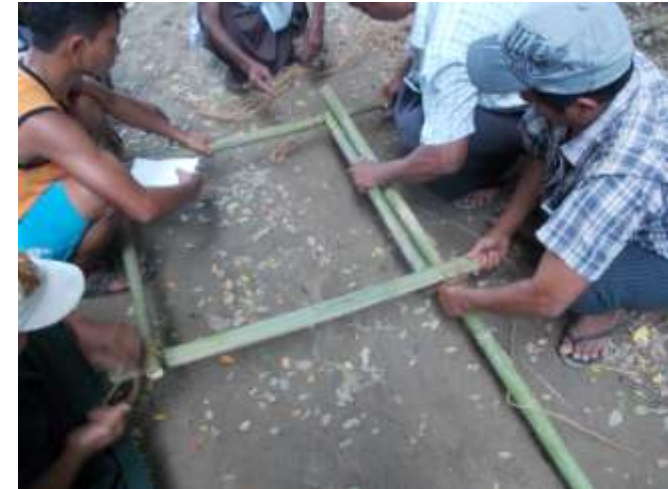
using a pre-cut 2ft 6in baton to set the frame square
