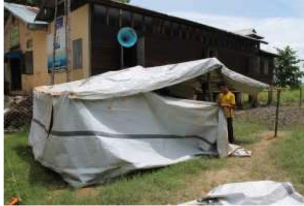
Halfway point; this is in fact the double elevated shelter that the emergency shelter can be upgraded to.
