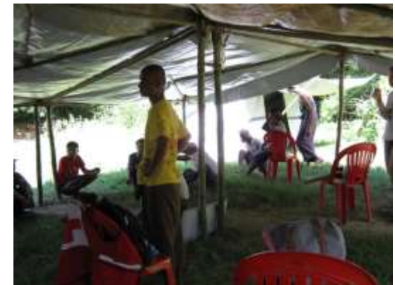
Double support poles for additional security
