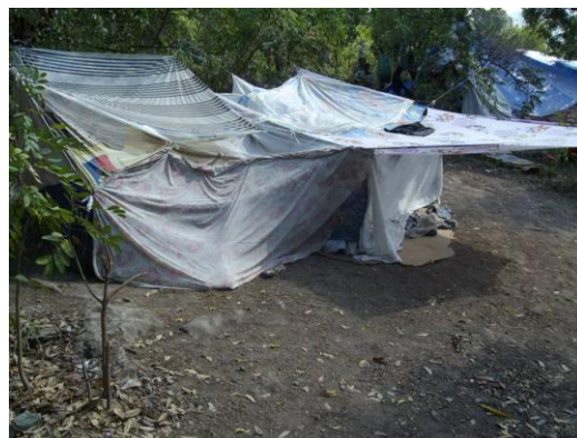
Figure 7; A shelter in post earthquake Haiti made from old bed sheets. A tarpaulin and frame could provide much more comfort and security than this type of shelter.(Photograph by Shaun Halbert)
