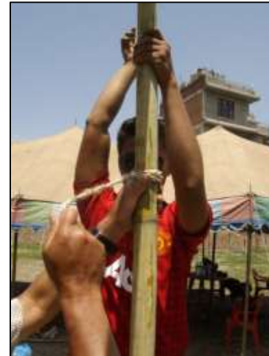
Tying a sliding knot
