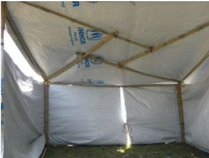
Effective tarpaulin support in the middle where needed most
