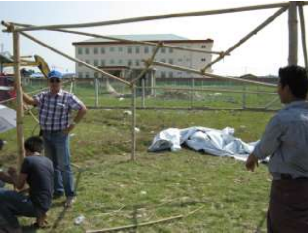
Frame complete and ready for tarpaulin attachment
