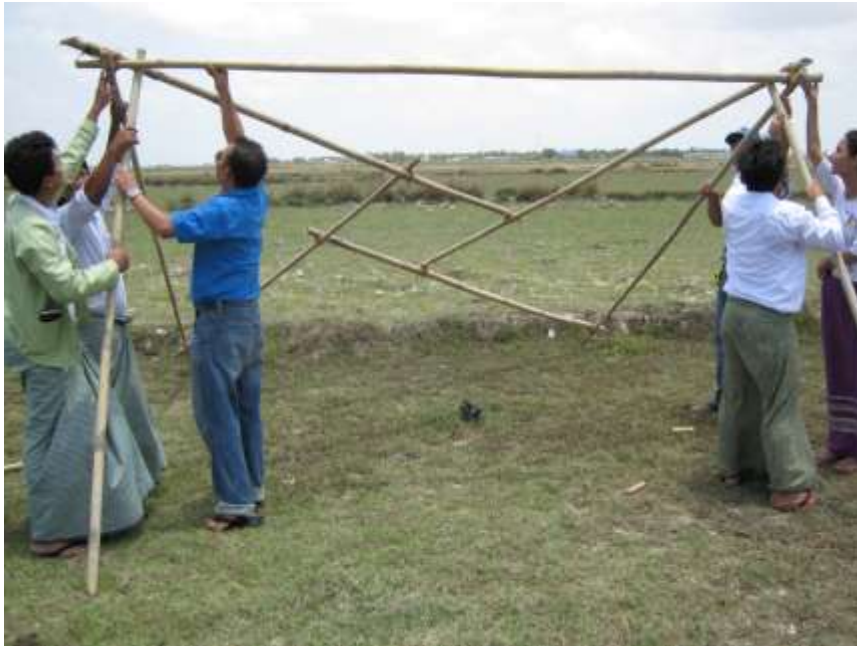
Support posts positioned inside frame
